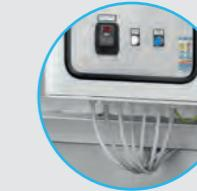
Electric panel with PLC installed on board and electric connections for all the electromechanical components placed in stainless steel ducts.
