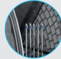
Electric level sensors for backwashing pump activation.
